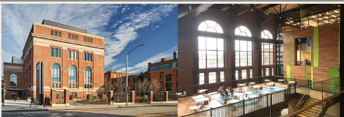
Post-rehabilitation exterior view
