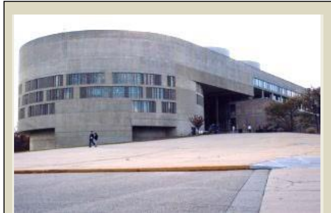
Unlike CCRI's Knight Campus in Warwick, many notable examples of post-World War II "modern" architecture in Rhode Island remain to be documented and registered.
